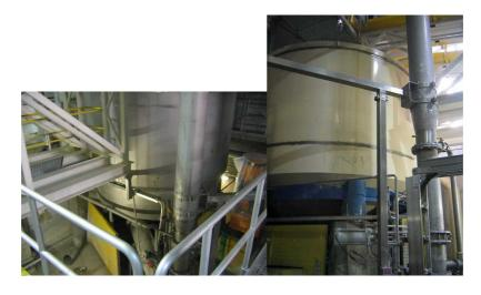
1 x Escher Wyss Pulper 20m3 with drive motor 160kW and short conveyor belt
